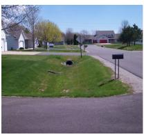
weathering, are washed from roadways by rain water. Ditch vegetation helps to trap these substances, and reduce flow rates, promoting settlement of solid particles and preventing them from entering the natural waterways.
