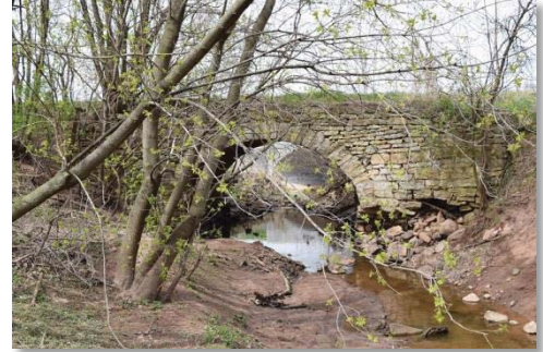
Allison Drive Bridge
