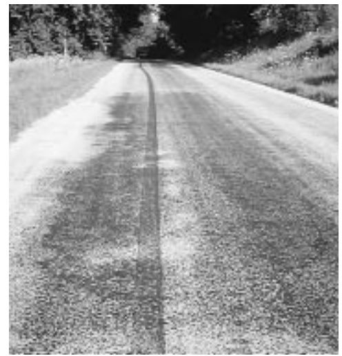
▼ Moderate flushing.
