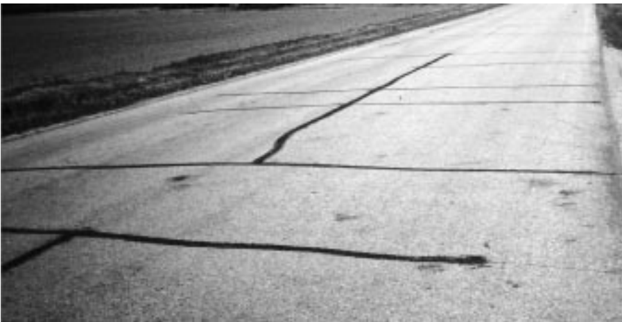
▼ Open crack, 1/2" wide; adjoining pavement sound.
