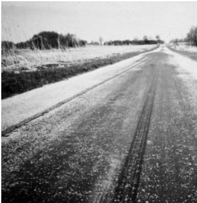
▼ Severe flushing.
