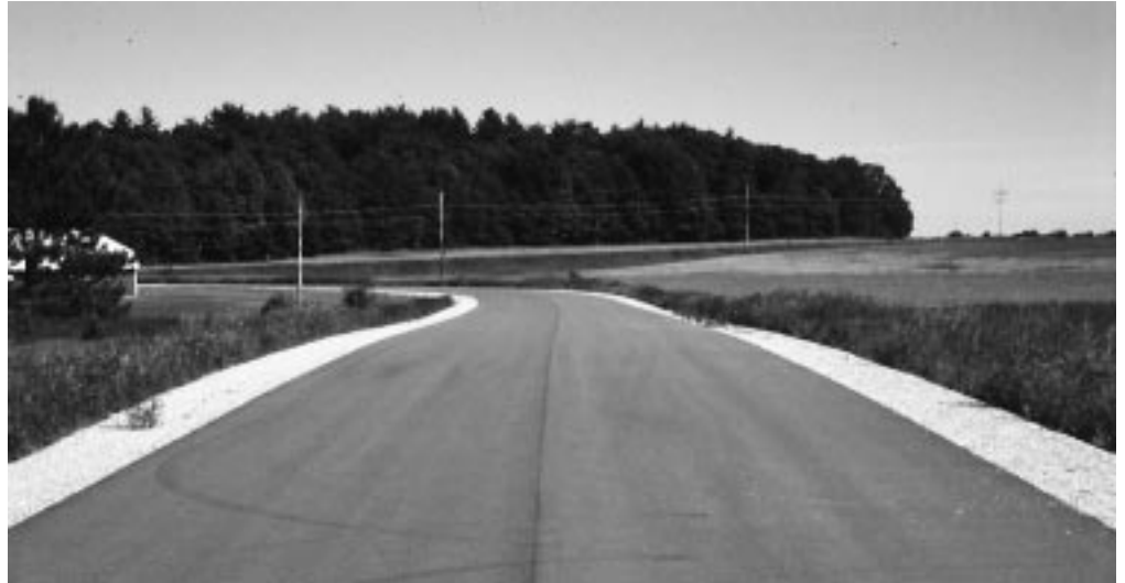
▶ RATING 10 New construction.
