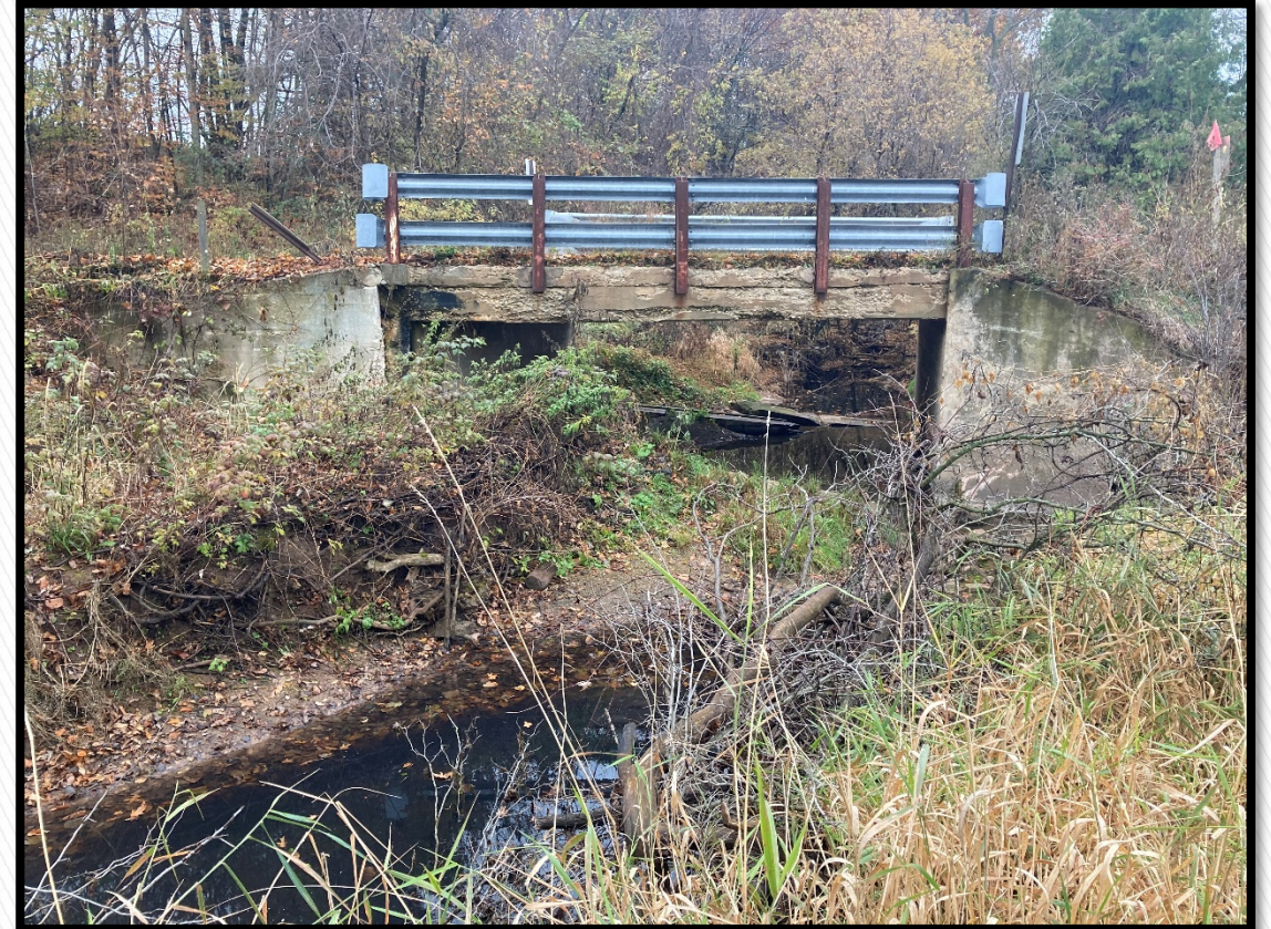
View of the current Branch of Plum Creek Bridge, looking west.
