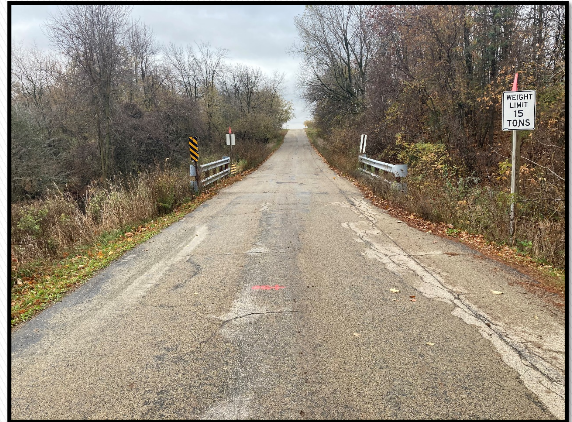
View of the current Branch of Plum Creek Bridge, looking south.
